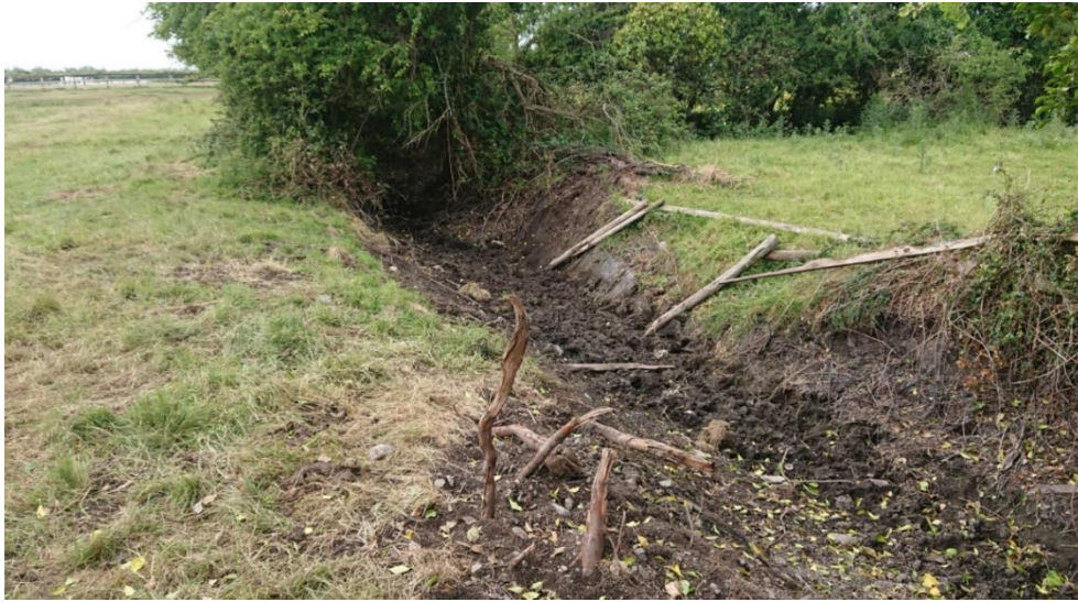
Figure 4-4: Old Ditch network post installation of Phase 1 relief ditch
