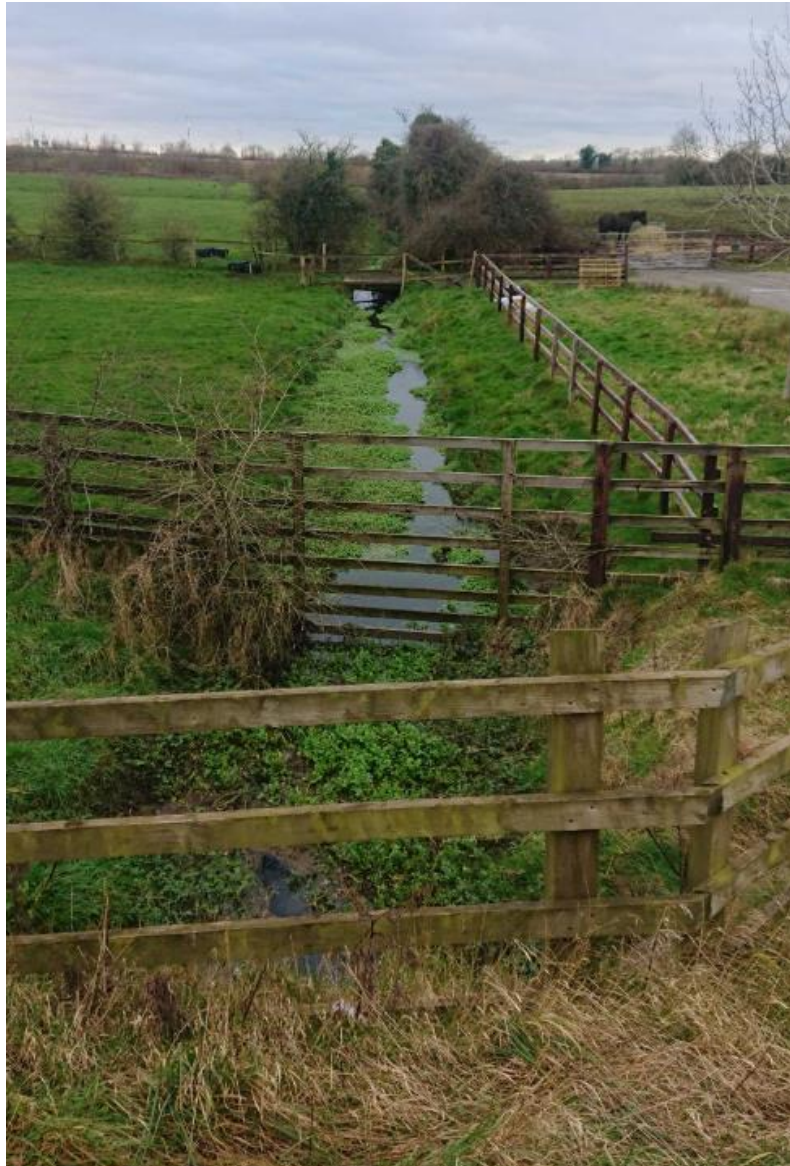
Photo 2: Skane River West of the R125 embankment
