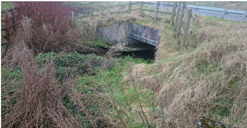
Photo 1: Existing Skane River Culvert under the R125 - looking west
