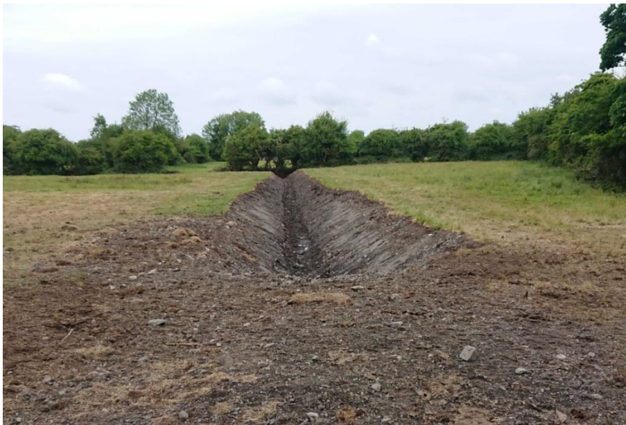
Figure 4-5: Phase 1 relief ditch
